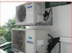
Install, Service & Repair Aircon
