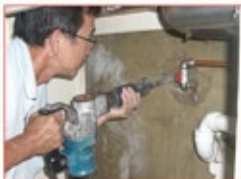
Repair Pipe Leaks Install Sink, Basin ...
