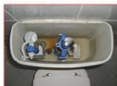
Repair Flush, Float, Change Toilet Seat
