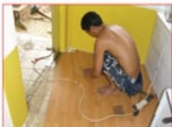
Install New Panel & Parquet Flooring...
