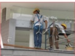
Minor & Major Repairs, Renovation...
