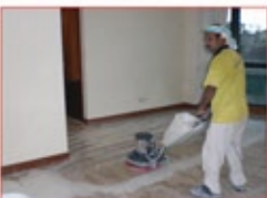
Polish Marble Floor & Vanity Grind & Varnish Parquet
