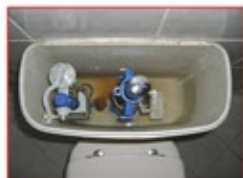
Repair Septic Tank Systems, Toilet Bowl...
