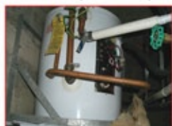
Repair & Install Storage Water Heaters...
