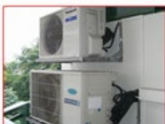
Service & Repair Aircon, Install New Aircons...
