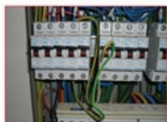
Repair Power Trip, Sockets, Switches,
