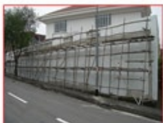
Painting, Cleaning, Water Proofing...
